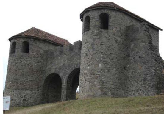
II.2 Porolissum camp gate (both reconstructed)
