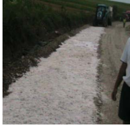
Road structure before recycling with fiber dispersion.
